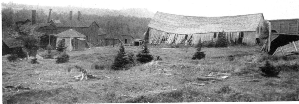
Old briquetting and smelting plant. Bog Manganese deposit, Dawson Settlement, N.B.
