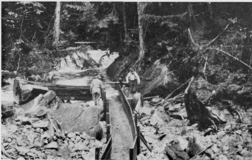
Main sluice-box, Potato Creek placers.
